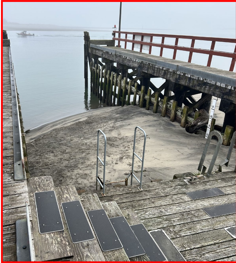
Sediment accumulation in the Station haul-out facility
